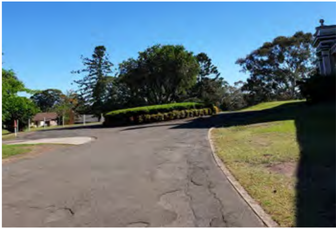
3. Carriageway Existing 19th century carriage way addressing Dunmore House to Dunmore Street. Several specimen trees are evident from 1943 aerial which remain today.
