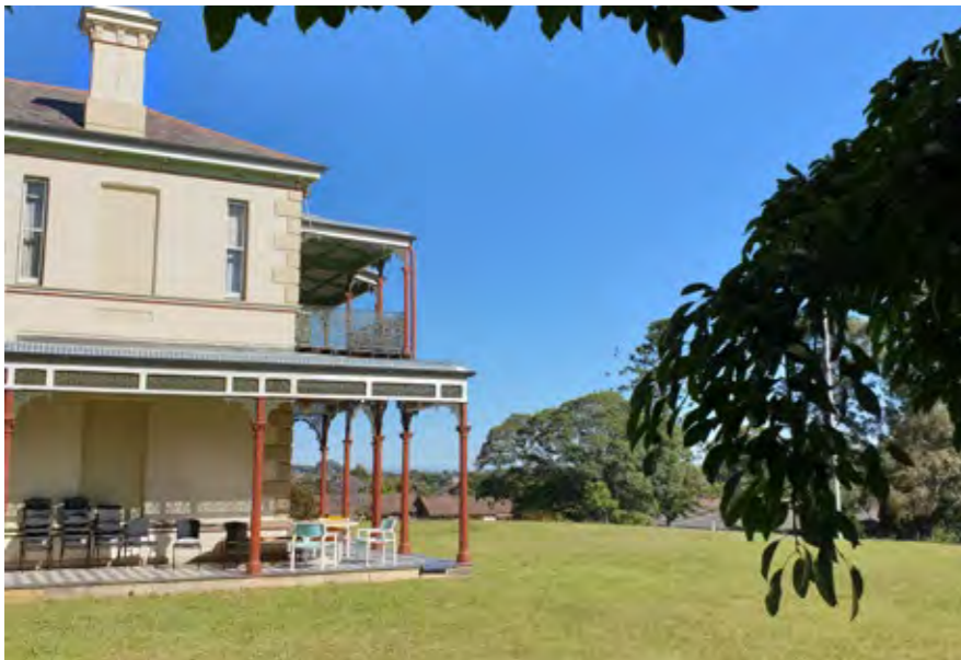
View of Dunmore House looking west
