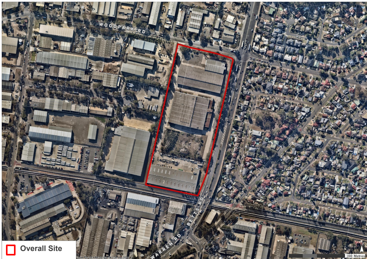
Figure 1 – The Overall Site (106-128 Woodpark Road, Smithfield)
