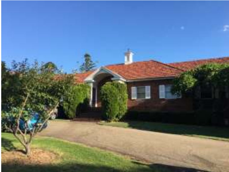
Figure 22: The managers cottage on the southern boundary.
