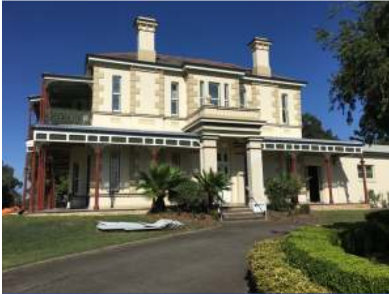
Figure 12: The western principal elevation of Dunmore House.
