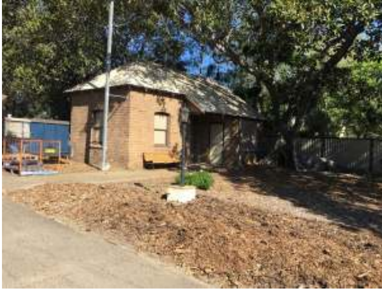
Figure 21: The managers cottage on the southern boundary.
