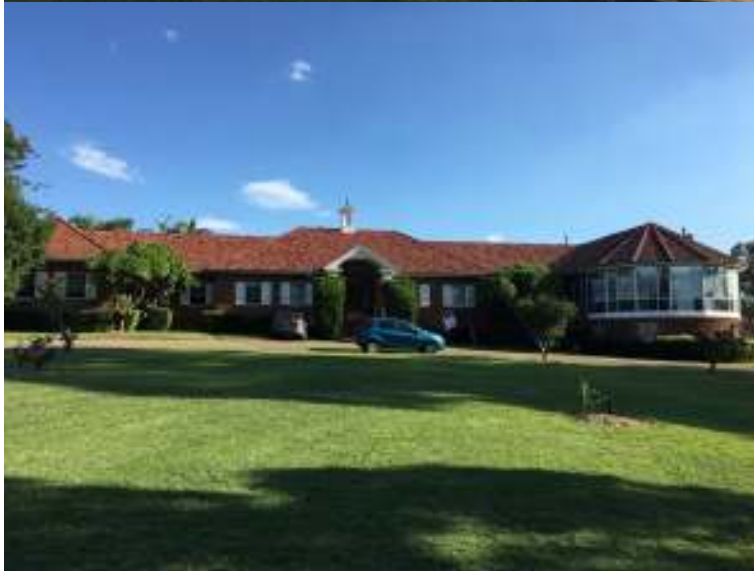
Figure 23: The managers cottage on the southern boundary.
