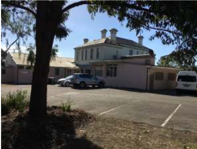
Figure 15: The eastern elevation showing later extensions.
