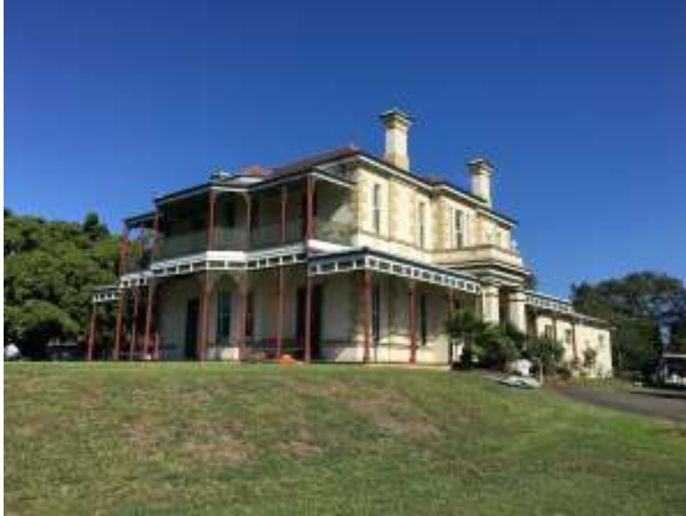
Figure 13: The northern elevation of Dunmore House which overlooks the open lawn area to the north.
