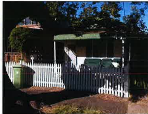
Figure 2: No.10 William Street (heritage item)
