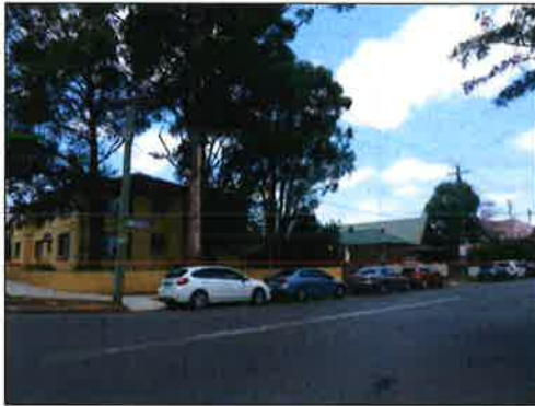
Figure 1: No.2 William Street, viewed from William Street
