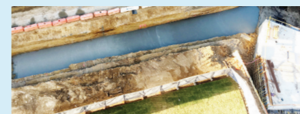
Merrylands Stormwater Upgrade
