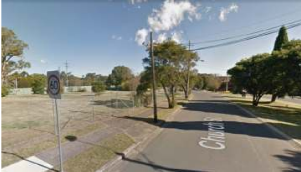
1 An unusable median strip is located to the north east of the site.
