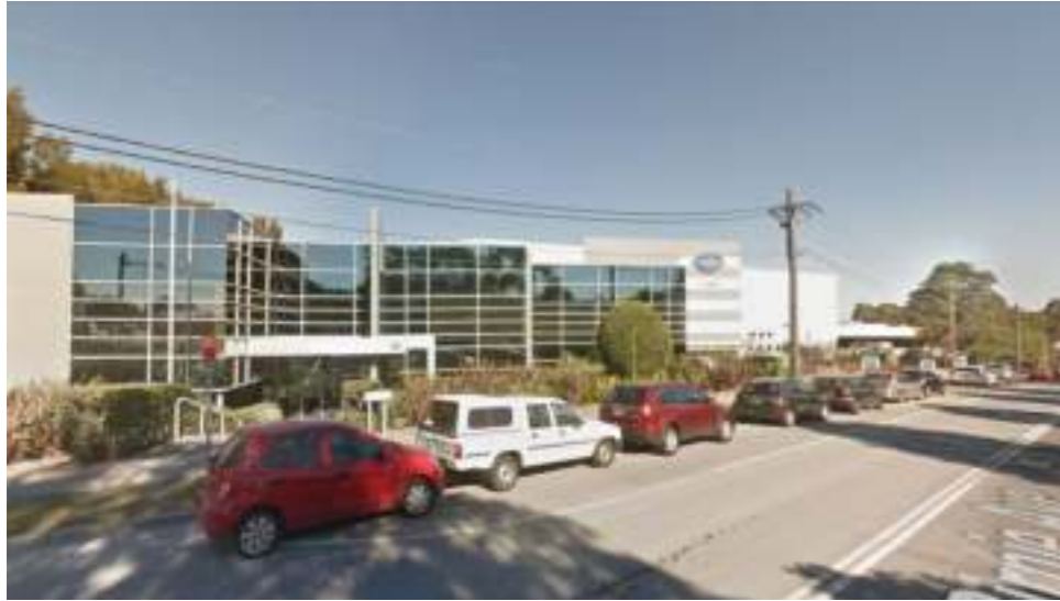
1 Lidcombe Industrial Area - Located east to the site.
