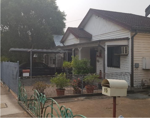
Picture 1 Single storey houses opposite the site on Church Street
