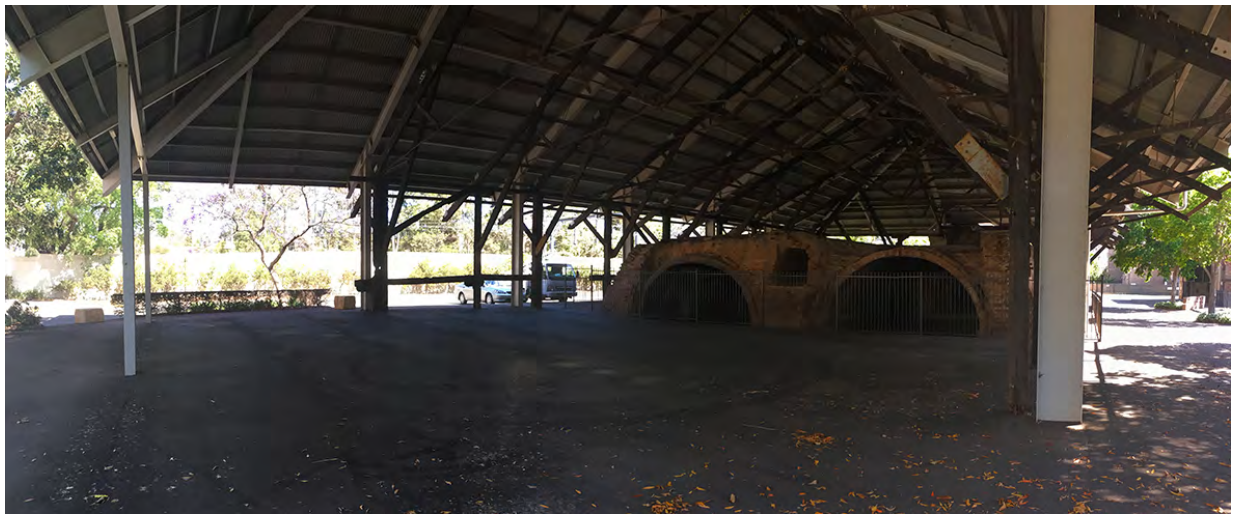
Building No 1 – shelter structure over remnant kiln fabric
