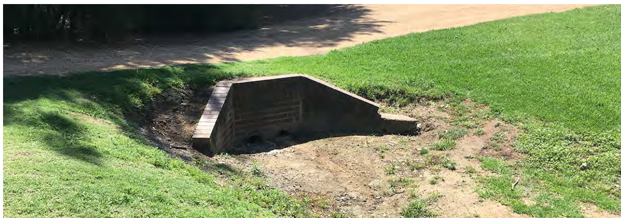
Where access crosses these swales they are provided with culverts.
