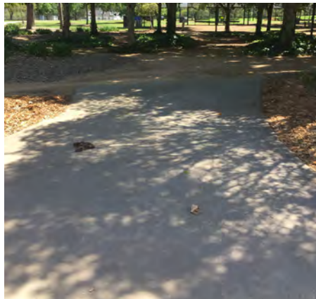
Existing concrete path links
