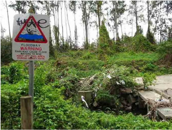
Flood warning sign at causeway
