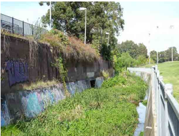
Channelled section of A'Becketts Creek
