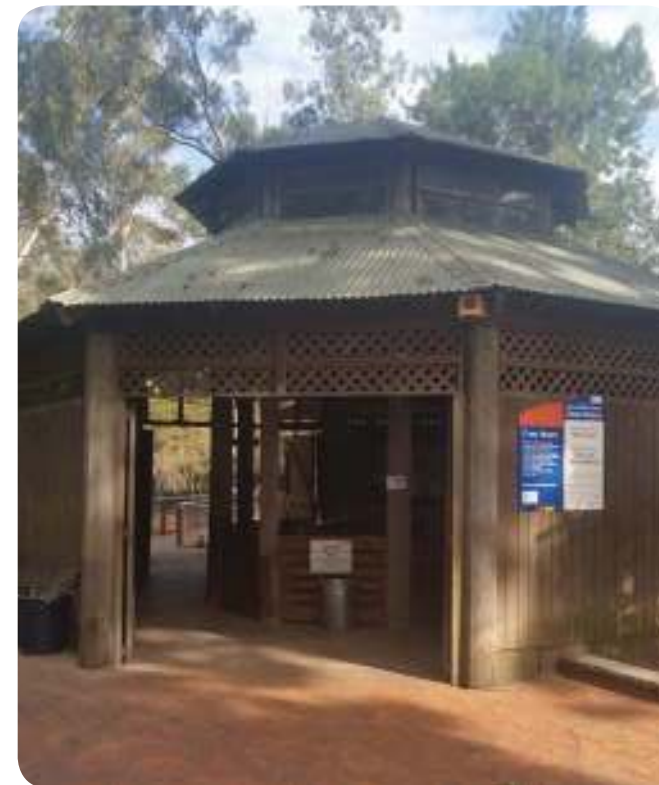
Entry structure to Fauna Park
