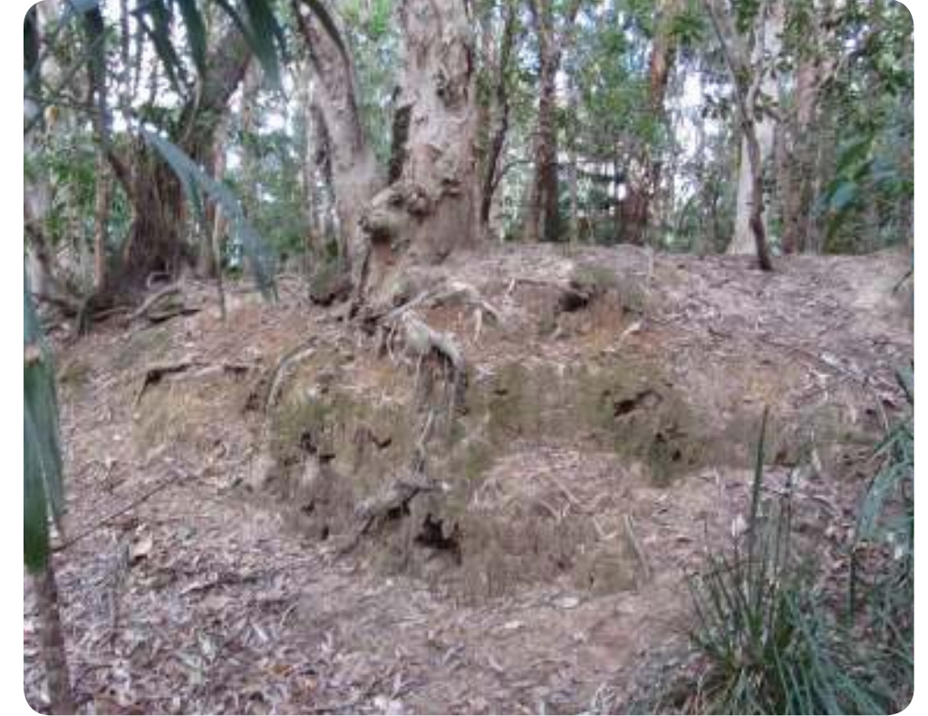
Eroded clay banks
