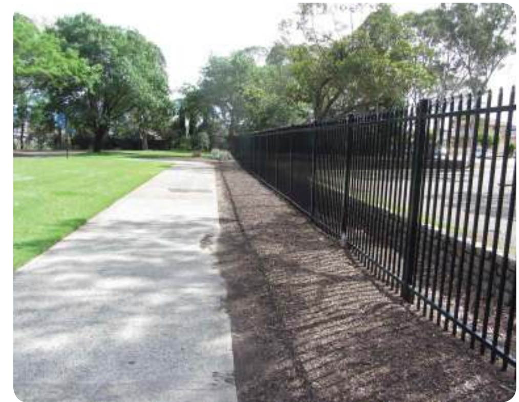
Chisholm Road boundary fence
