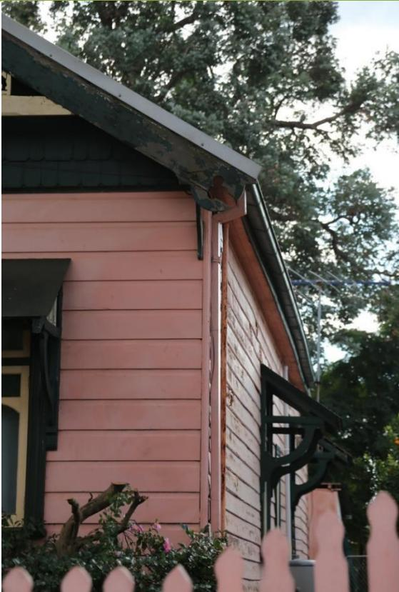
Detail of deteriorated timber to barge board.
