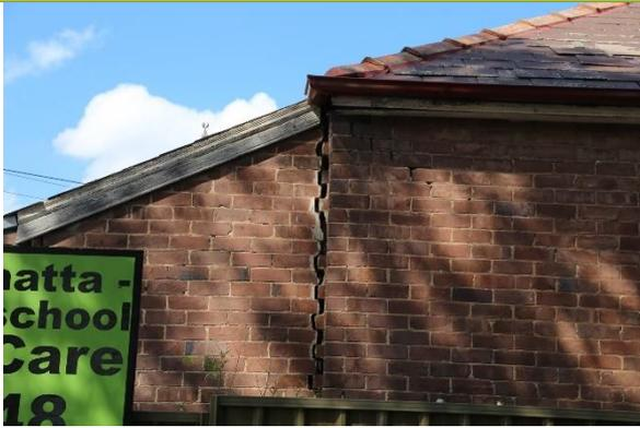
Detail of cracking in brickwork on the north elevation.
