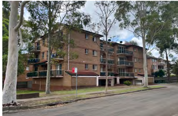
View of existing apartment buildings along Good Street
