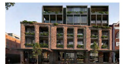
Fine grain detailing at the lower levels integrates well with the surrounding context (Cookson apartments, Redfern)
