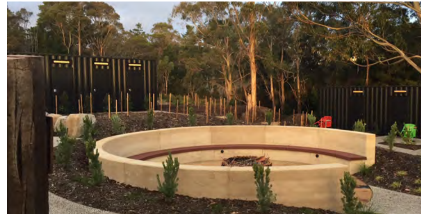
Rammed earth to showcase the geology and colours of local Country.
