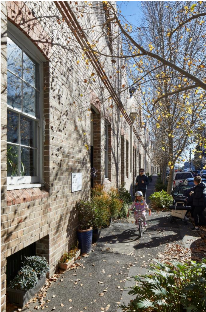
Figure 5 (above and top right) Retention of heritage facade at The Gantry by Bates Smart. Image: Martin Mischkulnig
