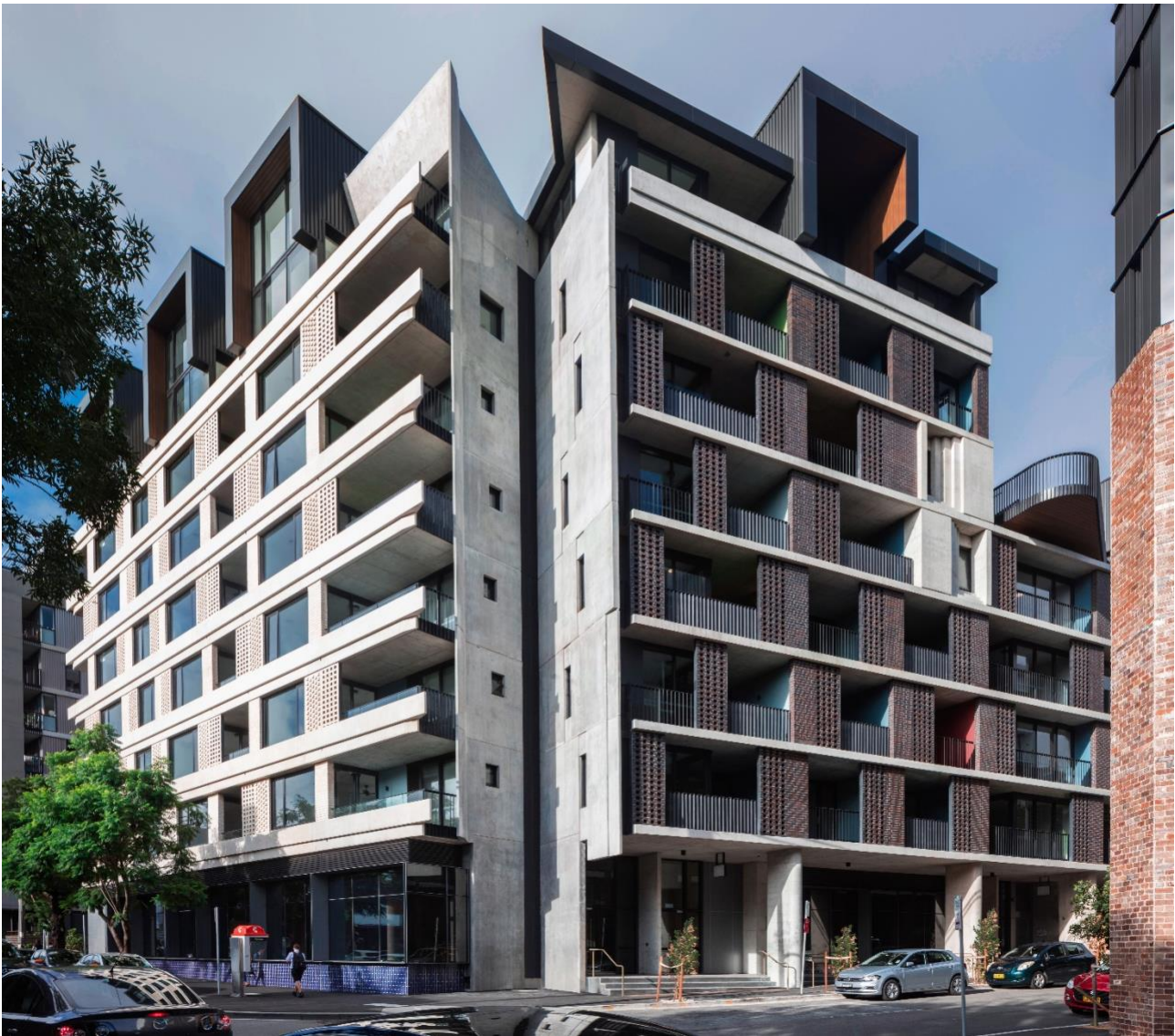
Figure 4 Active street frontage of Blackwattle Apartments in Glebe, by Turner. Image credit Brett Boardman Photography
