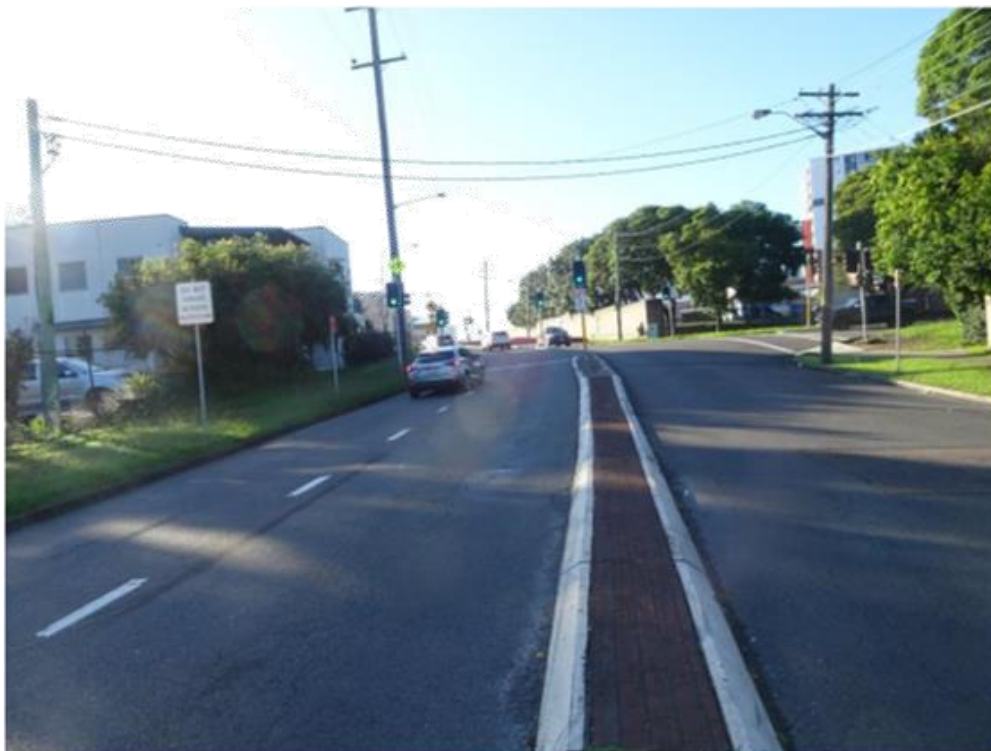
Figure 3A: Photograph of the South Parade at the signalised intersection
