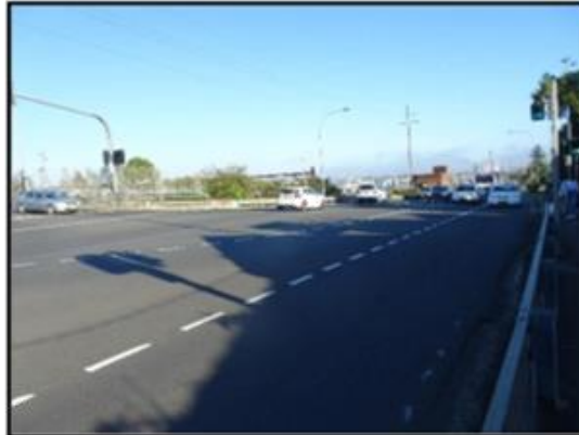
Figure 4f: Rawson Street from East to West
