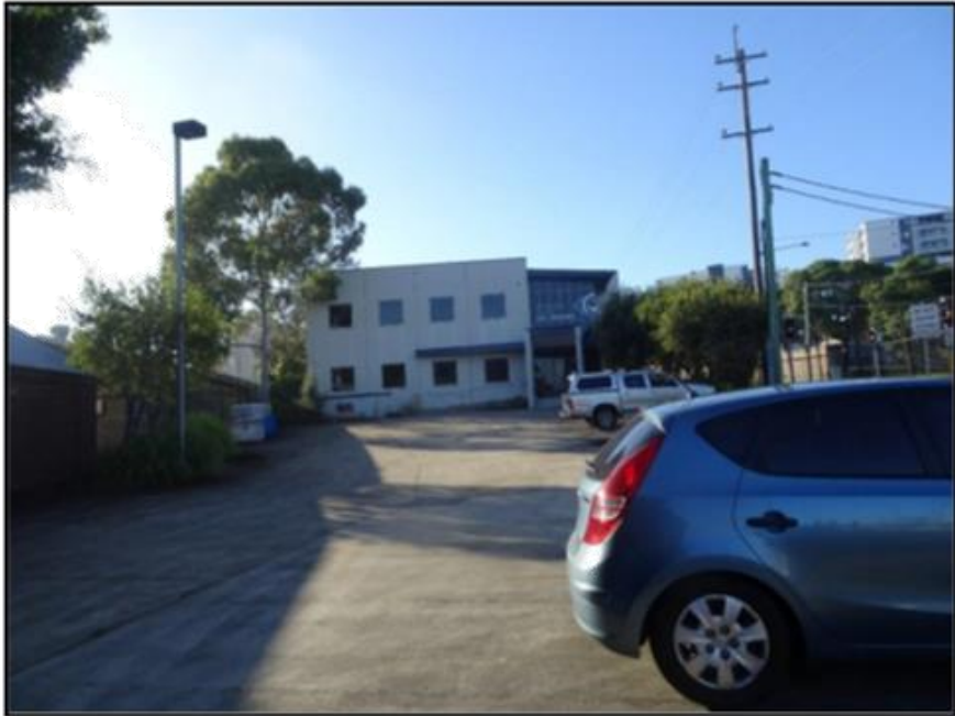
Figure 3: Photograph of the Site from South Parade
