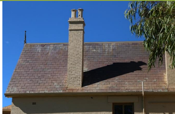
Detail of slate roof from Hawkesbury Road.
