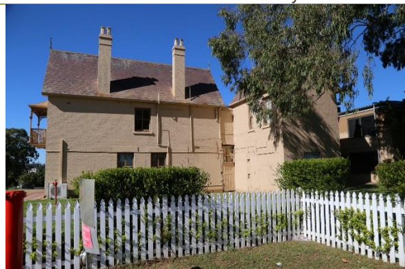
View of west elevation from Hawkesbury Road.
