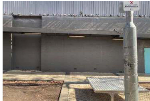
Looking to building facade to western edge.
