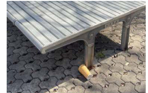
Existing permeable paving.
