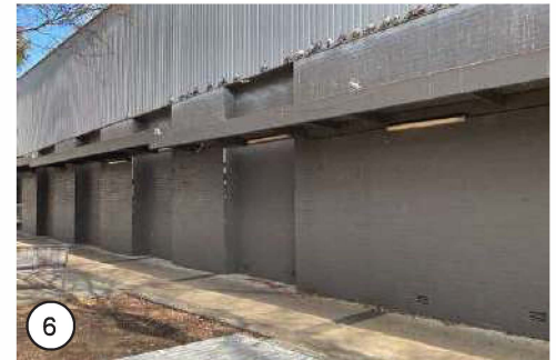
6 West wall facade of Guildford Plaza
