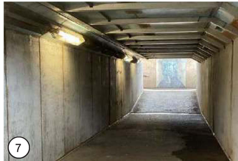
7 Guildford Station pedestrian underpass looking west
