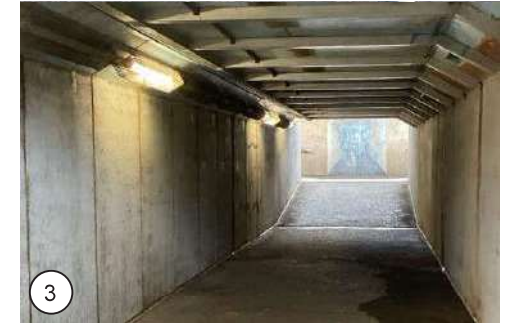
3 Guildford Station Tunnel
