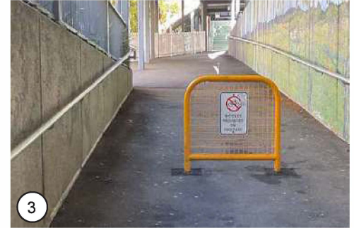
3 Guildford Station pedestrian underpass looking south
