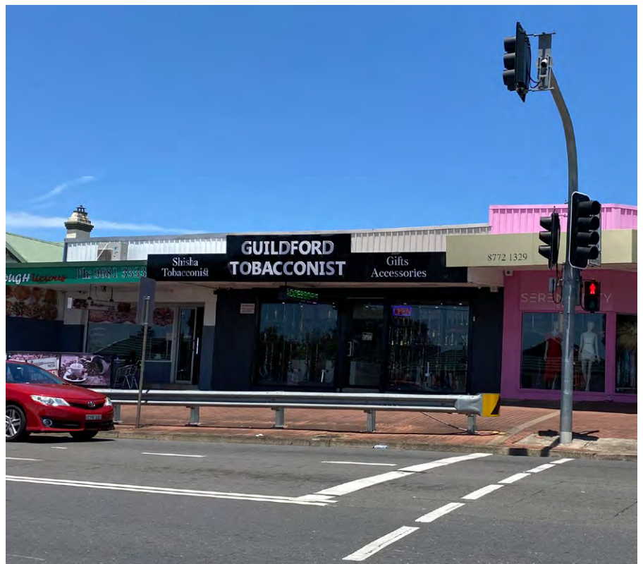
Figure 384 Signalised Pedestrian Crossing and Harsh Environment of the Road
