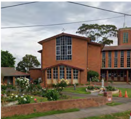
Figure 61 Holy Family Church (Source: Google Maps)
