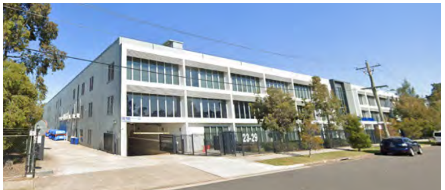
Figure 42 Large Commercial Building East of Duck River (Source: Google Map)
