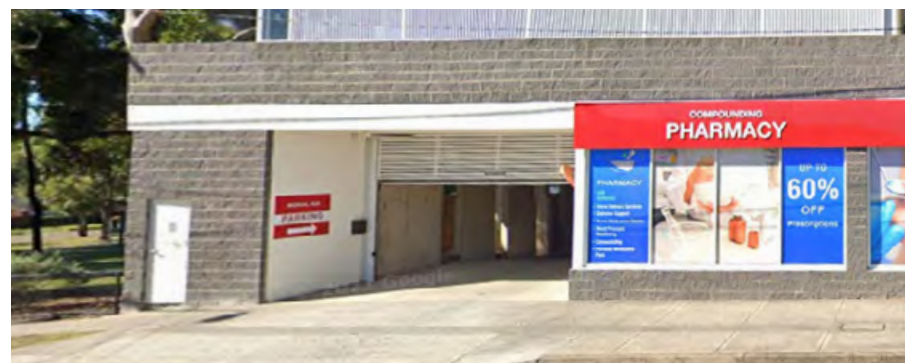
Figure 236 Underground Parking at the Medical Centre (Source: Google Map)
