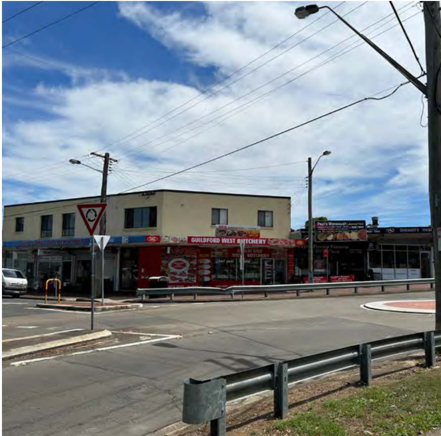
Figure 135 Safety Barriers and Worn Wooden Light Poles
