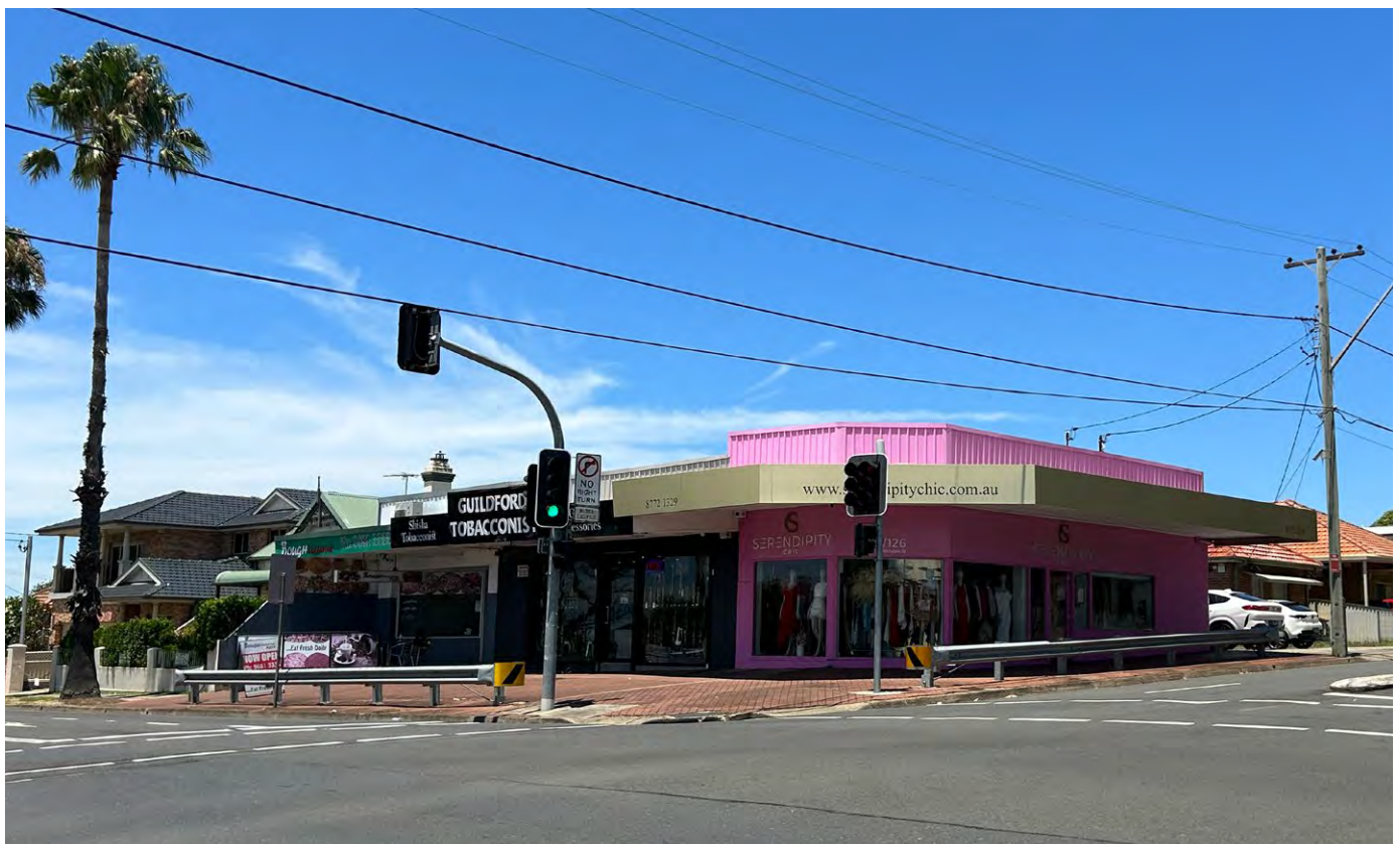
Figure 376 Hawksview Street Local Shops - View South-East from Hawksview Street
