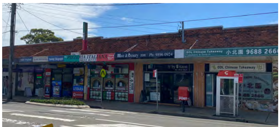
Figure 206 Unmodernised Shops along Old Prospect Road
