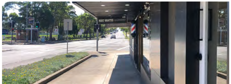
Figure 17 Shops awning - Looking East from Merrylands Road
