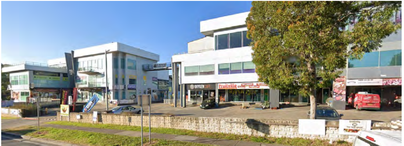
Figure 264 Buildings east of the Centre along Wellington Road in Poor Condition
