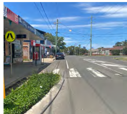
Figure 196 Pedestrian Crossing at Old Prospect Rd, West of Hampden Rd
