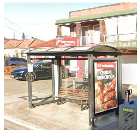
Figure 429 Sheltered Bus Stop at the Centre (Source: Google Map)
