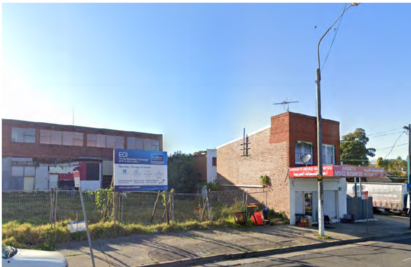
Figure 303 Footpath Condition (Source: Google Map)
