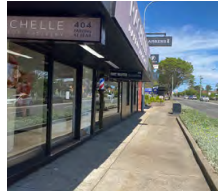
Figure 12 Existing Activity and Frontages - Looking West from Merrylands Road
