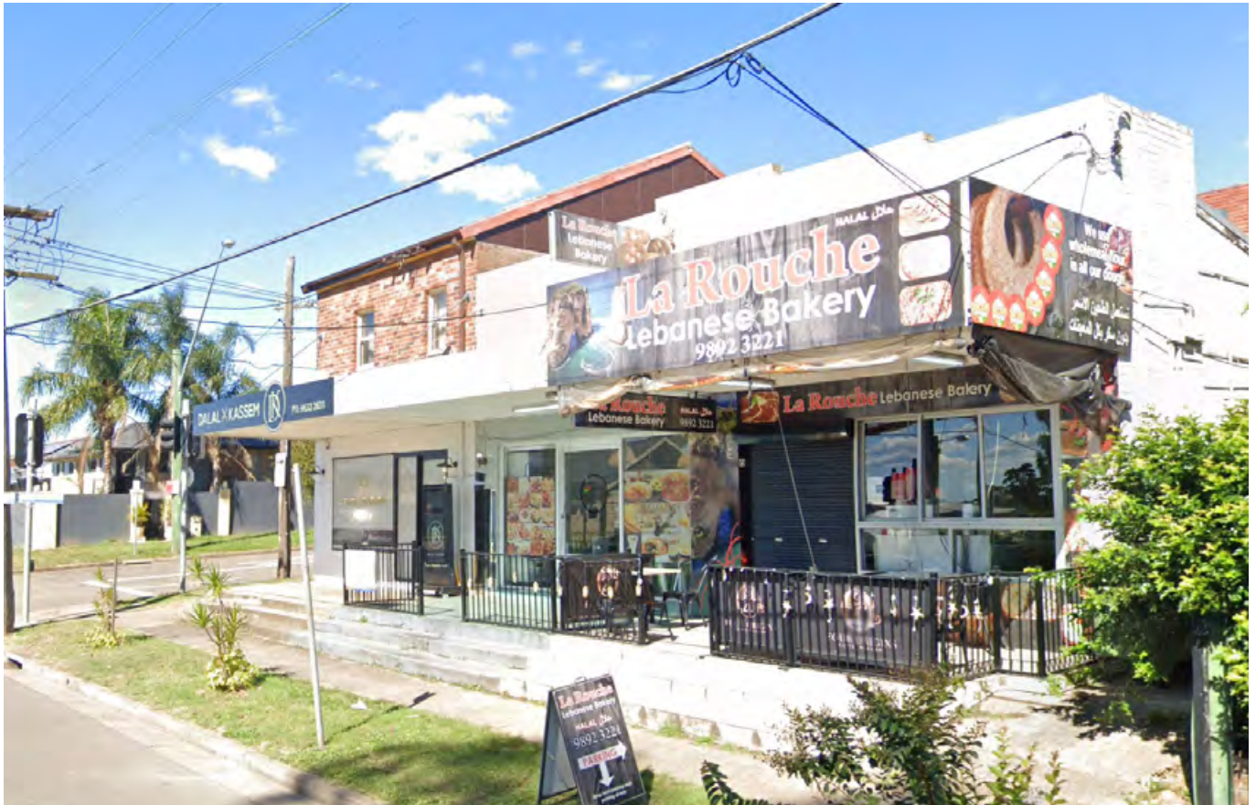
Figure 289 Built Form of Local Shops (Source: Google Map)
