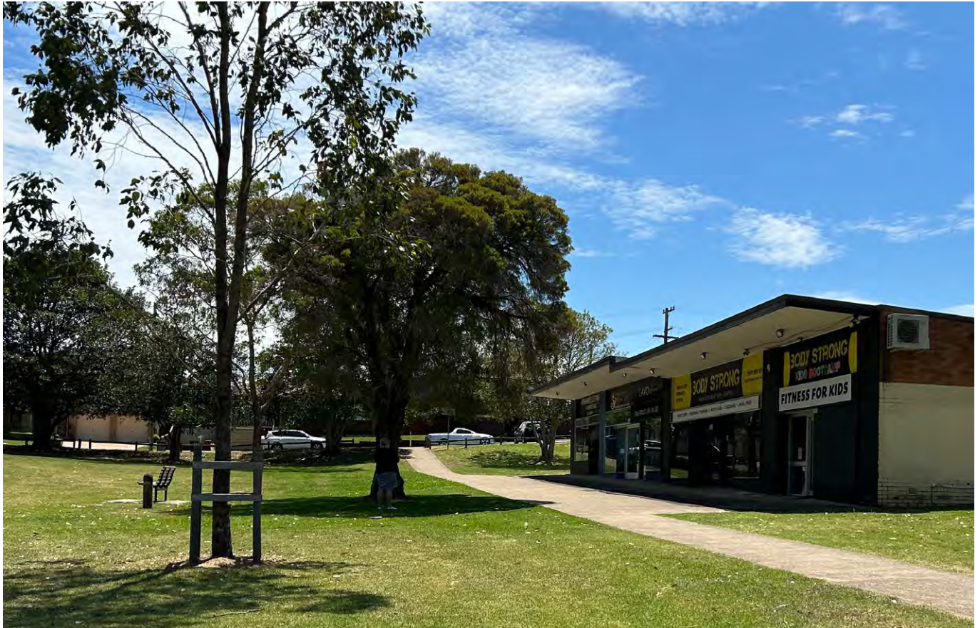
Figure 354 Renovated Building Frontage and Awnings
