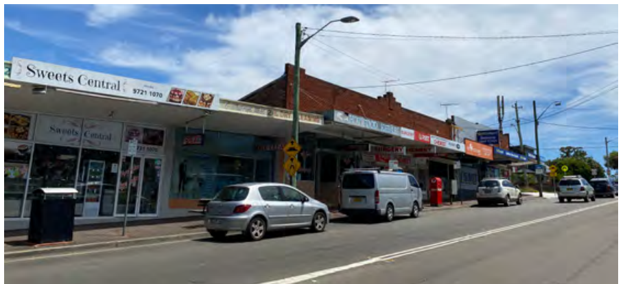
Figure 141 Single Storey Shops
