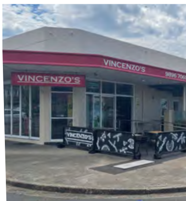
Figure 98 Refurbished Corner Italian Restaurant Building
