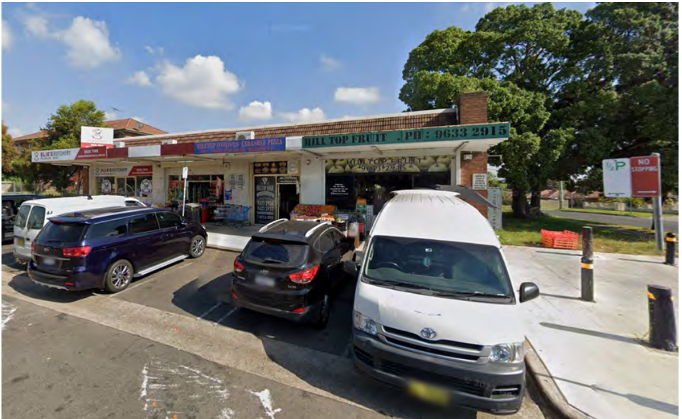
Figure 161 Local Shop View West at Coleman Street (Source: Google Map)
