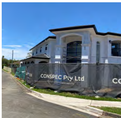
Figure 159 New Development under Construction
