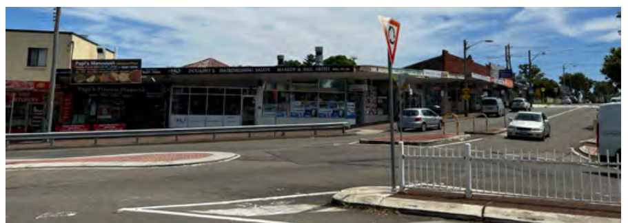
Figure 132 The Barrier along Guildford Road and Pedestrian Refuge at Intersection
