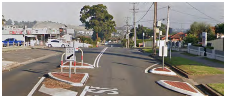
Figure 314 Pedestrian Refuge on Bathurst Street (Source: Google Map)
