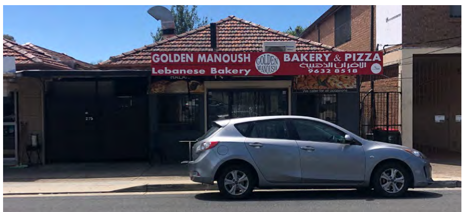
Figure 449 Single Storey Pizza Shop
