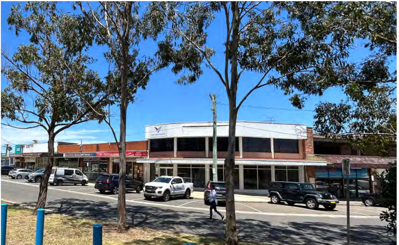
Figure 143 Local Shop View from Woodpark Reserve
