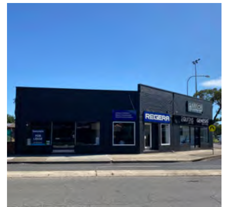
Figure 14 Example of limited landscaping - Looking North from Merrylands Road
