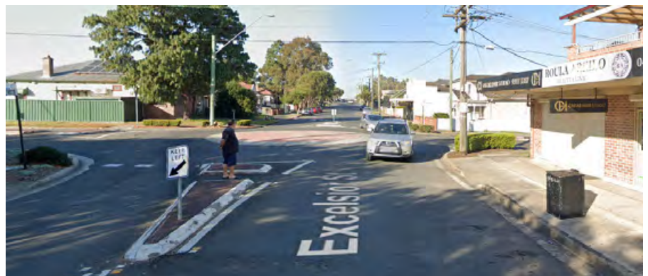
Figure 251 Pedestrian Refuge on Excelsior Street (Source: Google Map)
