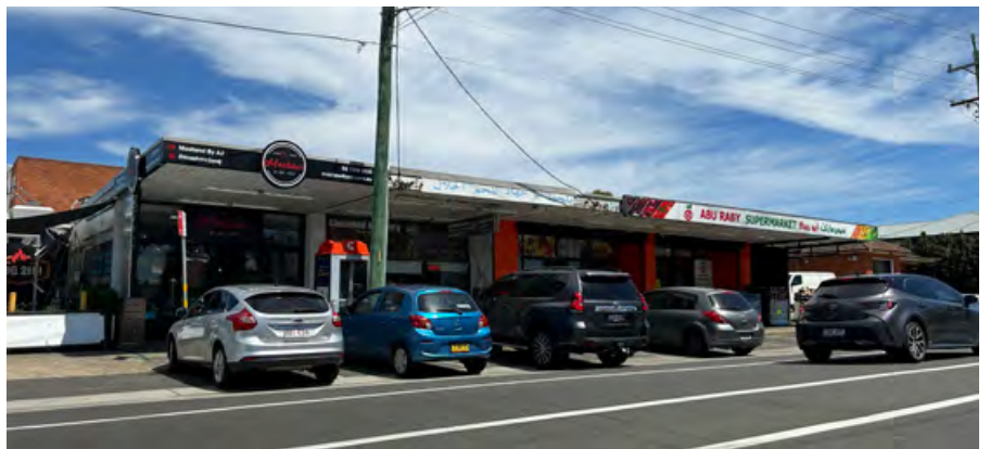
Figure 222 Single Storey Retail Shops
