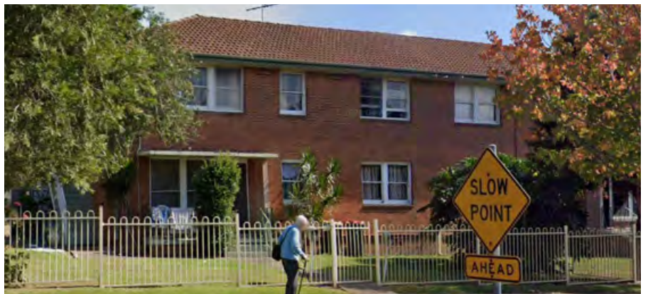
Figure 181 Two-storey Apartment Building Sitting Next to the Local Shops (Source: Google Map)
