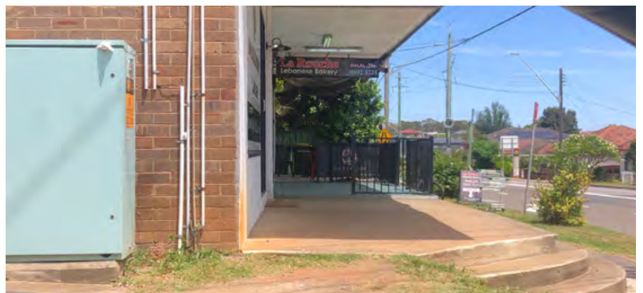
Figure 293 Shading Provided By Awning
