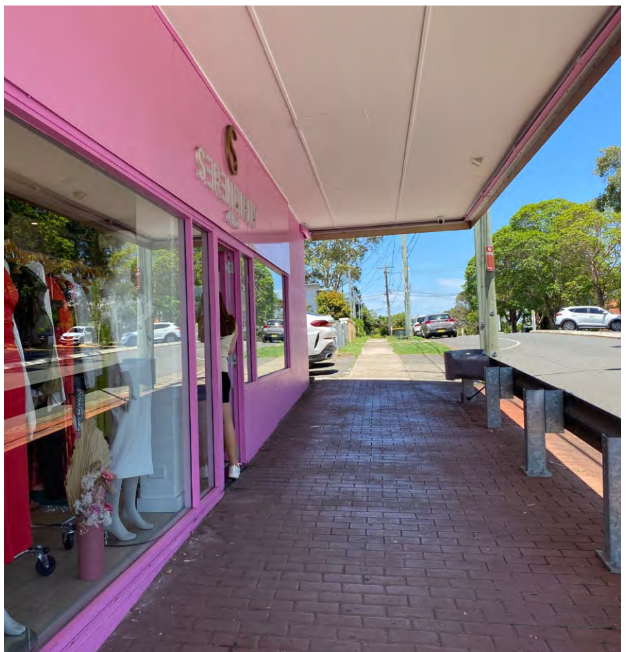
Figure 393 Awnings Providing Shading to the Footpaths
