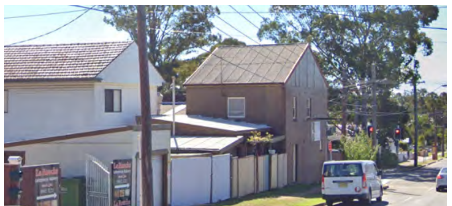
Figure 294 Two Storey Height Shop Top House Looking North from Blaxcell Street
