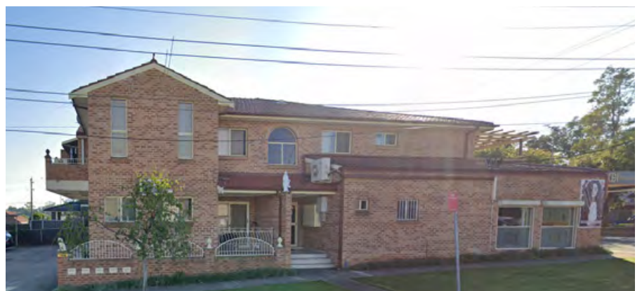
Figure 259 Residential Character of the Shop Top Housing along Farnell Street
