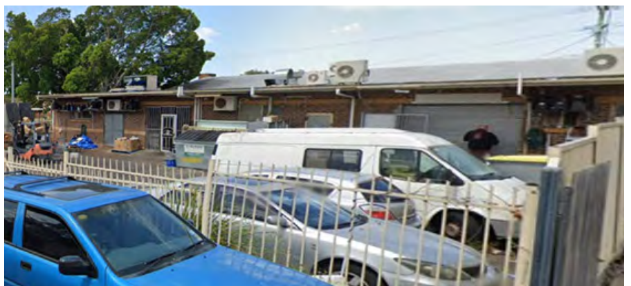
Figure 182 2-Building Condition, Looking East form the Rear-Laneway (Source: Google Map)
