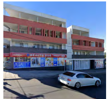
Figure 240 Mona Street sloping down towards east (Source: Google Map)
