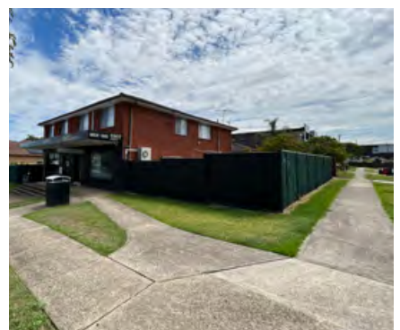
Figure 335 Ramp Access from Lucinda Road
