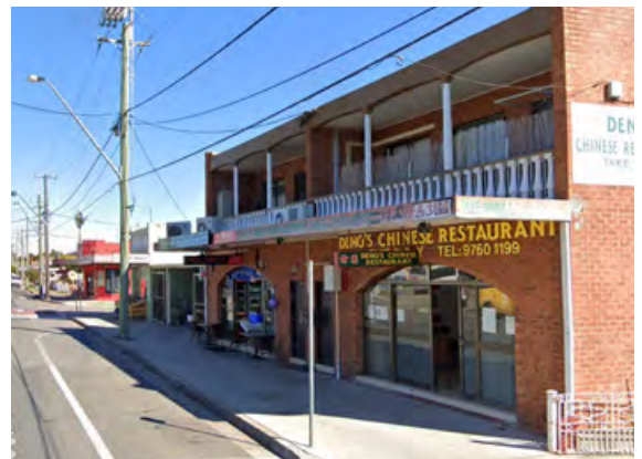
Figure 56 Example of the Condition of Awnings along Blaxcell Street
