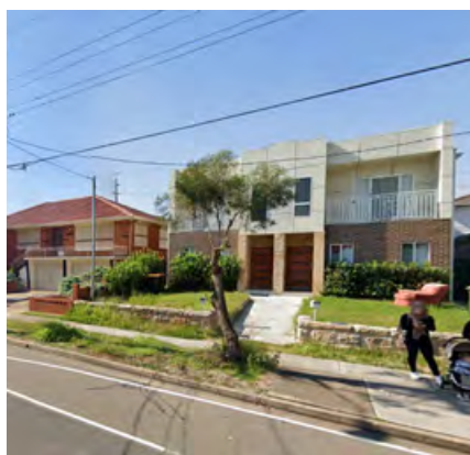
Figure 118 Low Rise Residential Buildings opposite the Local Shops
