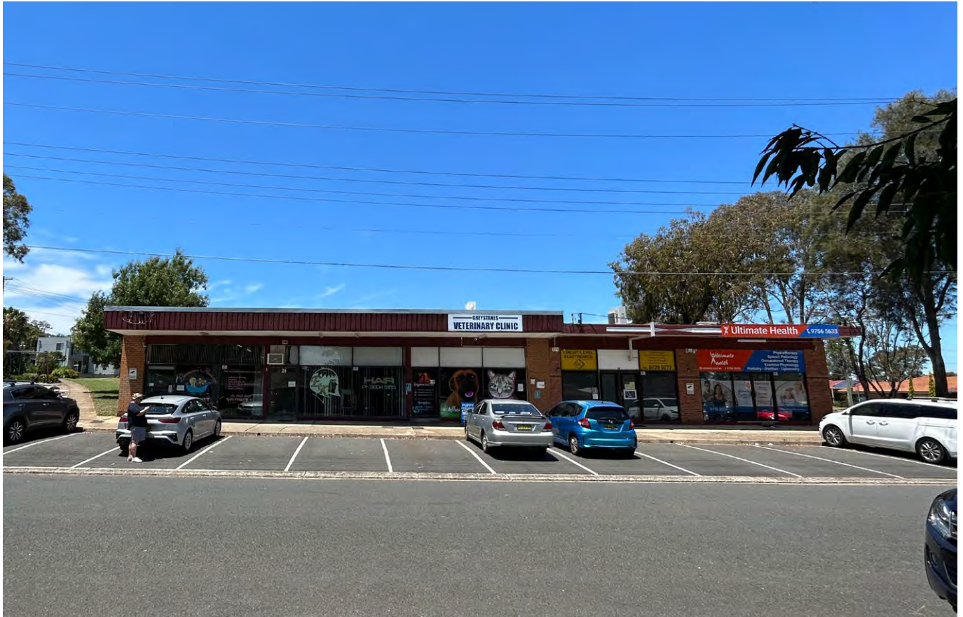
Figure 370 Convenient Access to Dedicated Parking Space in Front of the Local Shops
