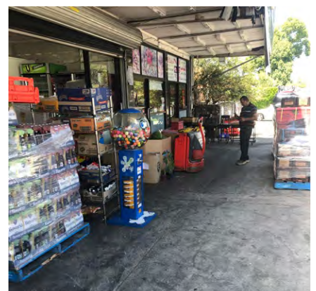
Figure 408 Condition of Footpaths in front of the Supermarket
