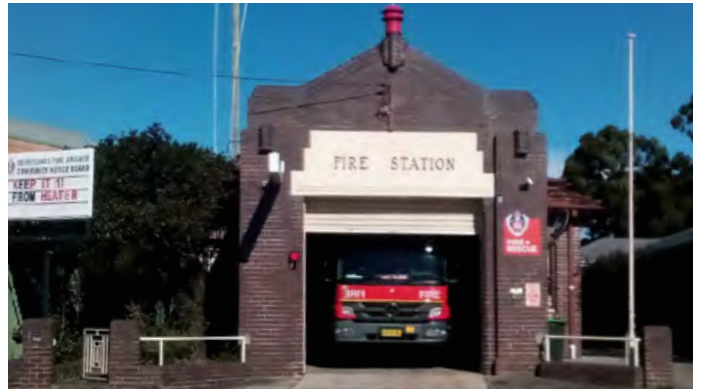
Figure 5 Fire Station Heritage Building along Merrylands Road ((Source: Google Maps)
