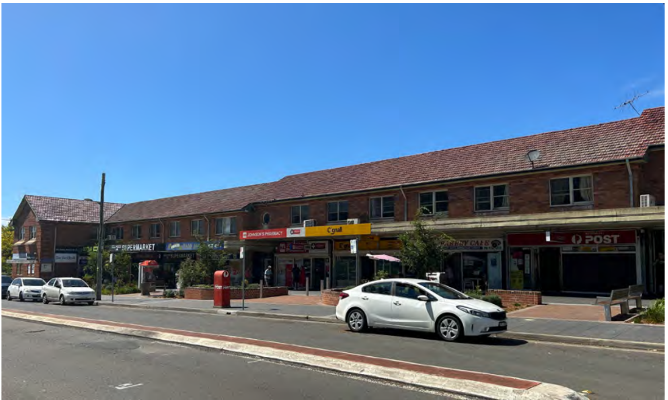
Figure 58 View South on Dellwood Street of Local Shops Cluster
