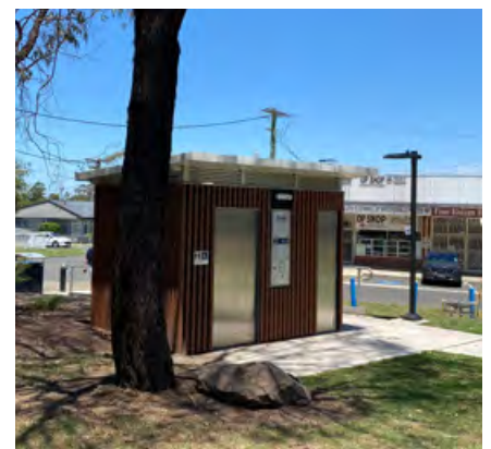
Figure 156 Smart Toilet at Woodpark Reserve
