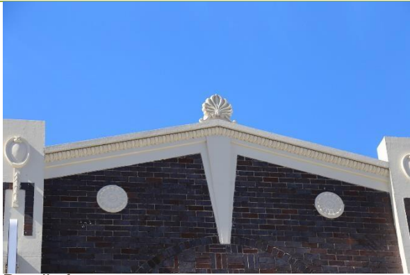
Detail of parapet.
