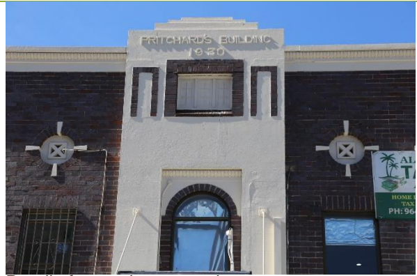
Detail of central parapet pier.
