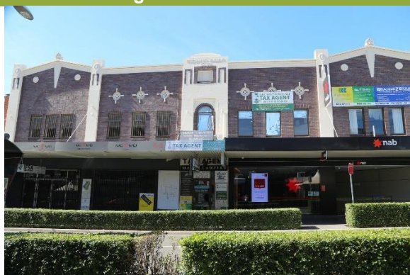
Façade of Pritchard's building
