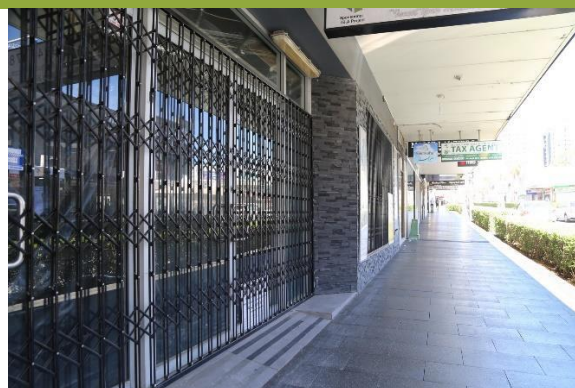
View along ground floor of shops.
