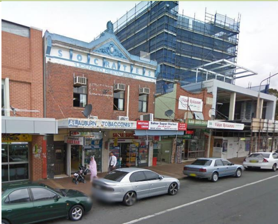
Google Streetview c.2009 showing adjacent land under construction in the background.
