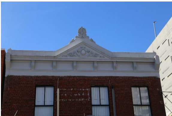
Detail of parapet on 60-62 Auburn Road.
