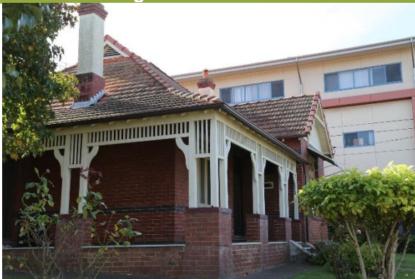
Verandah of residence.
