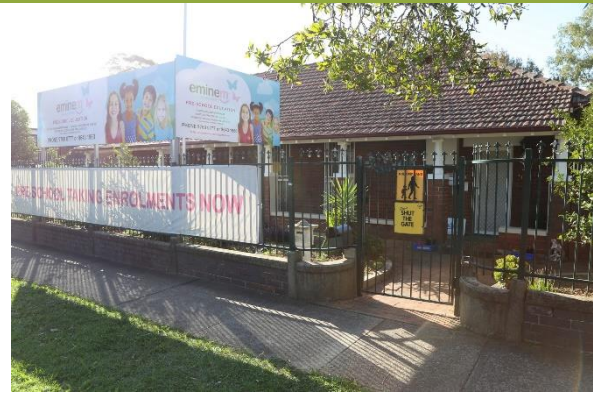
View to front entrance gate.
