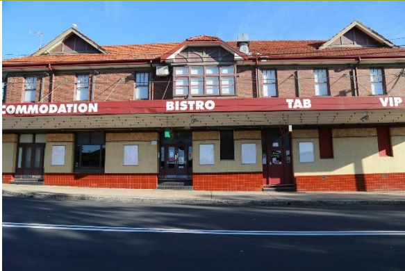
Melton Hotel, elevation along Station Street.
