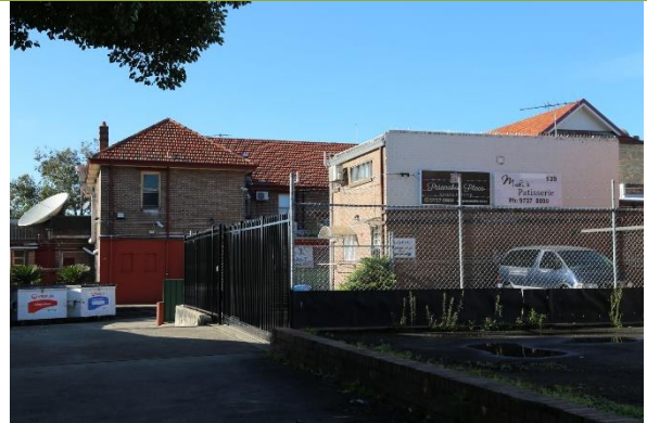
Rear of Melton Hotel.
