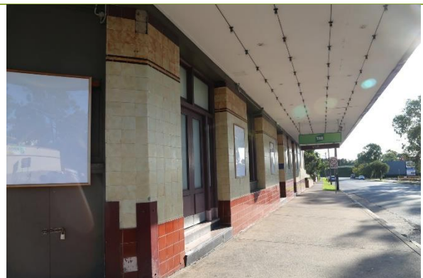
View along Station Road.
