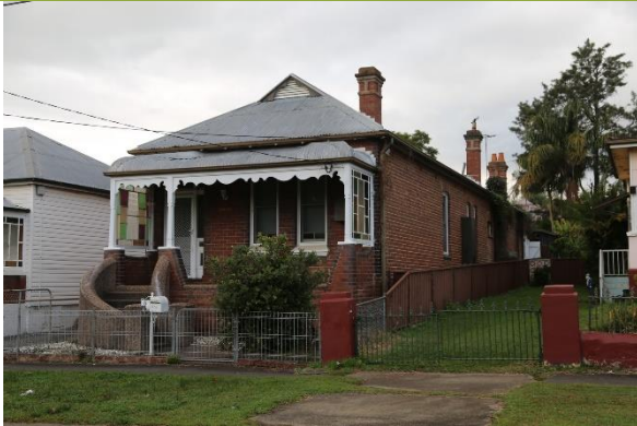
View to north and west elevations.
