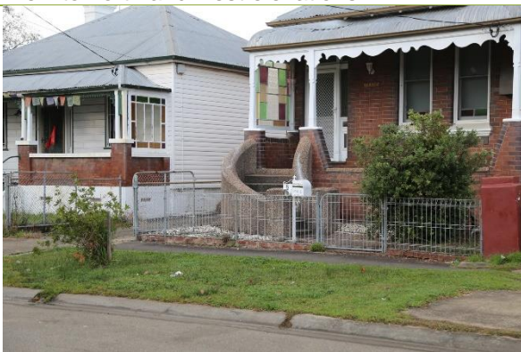
Detail of front verandah stairway.
