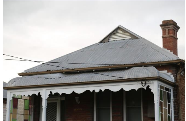
Detail of roof
