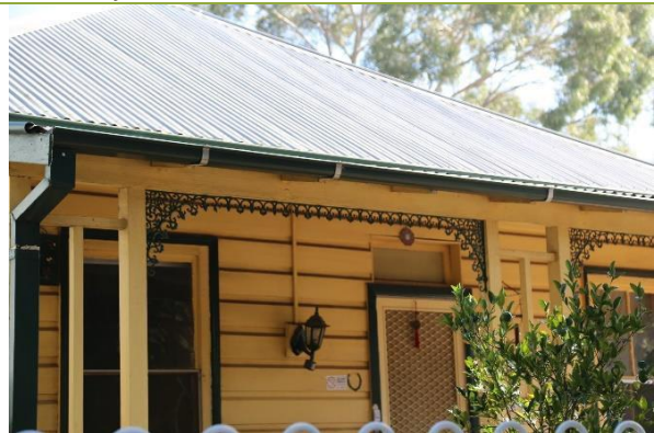
Detail of verandah.
