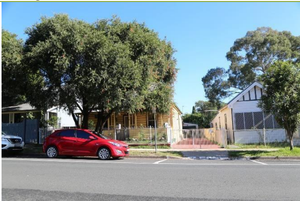
Overview of cottage.
