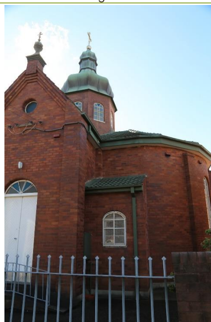
Detail of Church façade.
