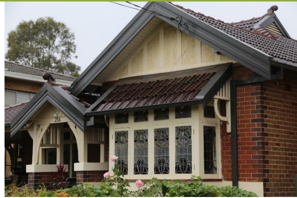
Detail of projecting wing.
