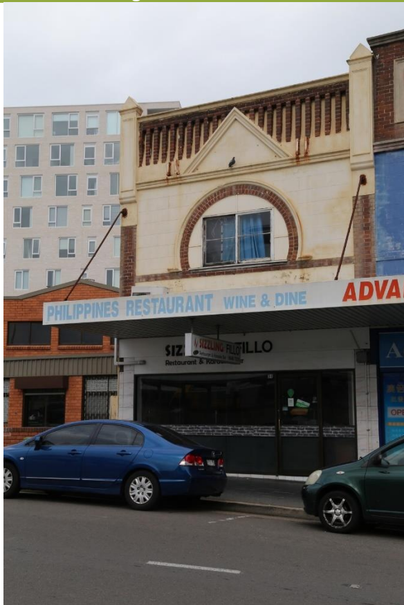
36 Railway Street, Lidcombe
