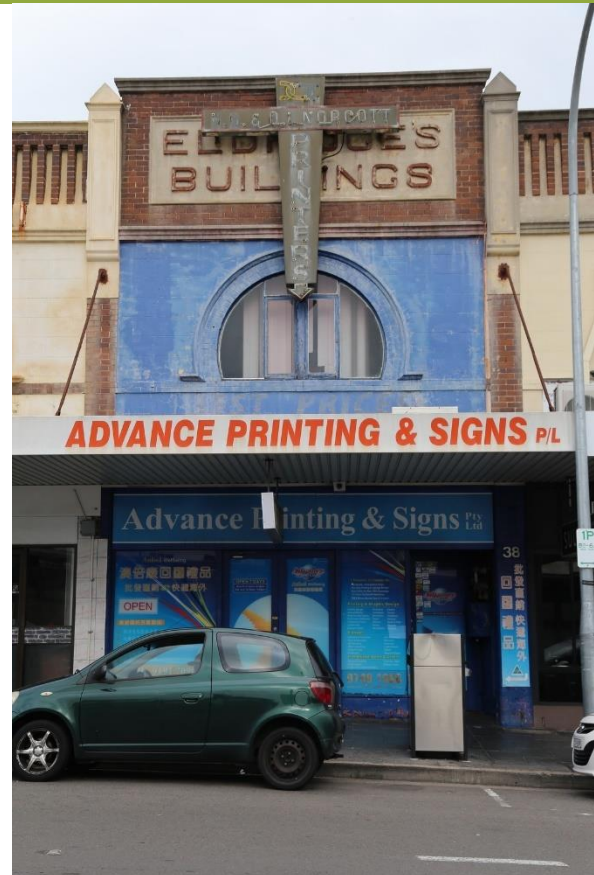
38 Railway Street, Lidcombe
