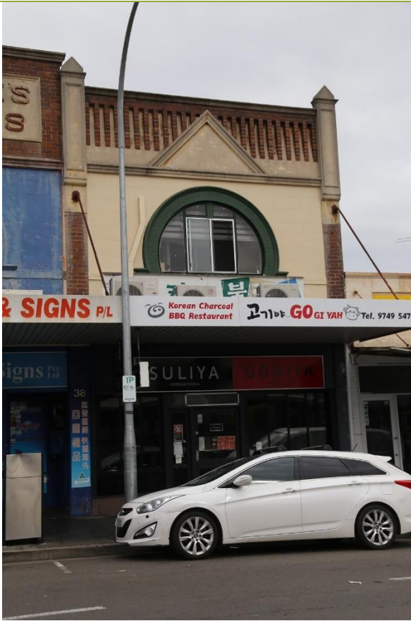
40 Railway Street, Lidcombe
