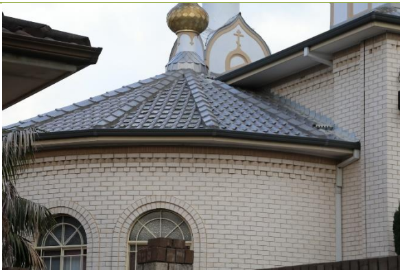
Detail of nave.
