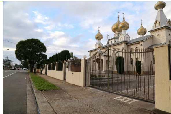
View of Church along Vaughan Street.
