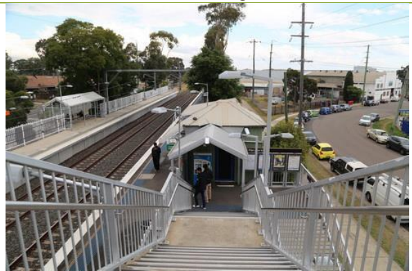
View northeast from Footbridge to Platform 1.
