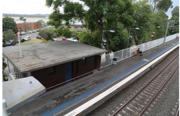
View southeast from footbridge to Platform 1.
