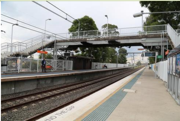
View from Platform 2 southeast to Platform 1.
