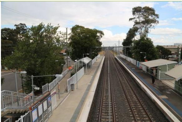
View northeast from Footbridge
