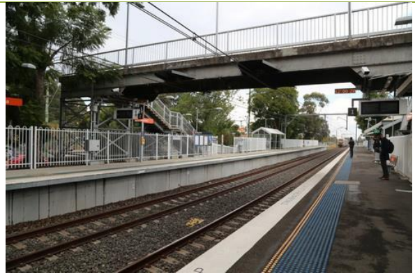
View of footbridge from Platform 2.
