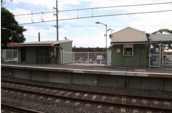
View to Platform 1 station elements
