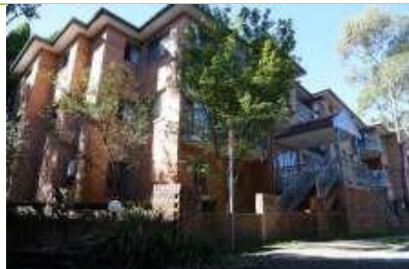
View to rear development fronting Thomas May Place.
