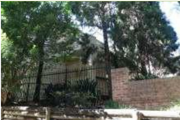
View of rear elevation of Inter-War apartment block.
