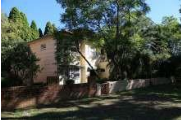
View of front façade, fronting the Domain.
