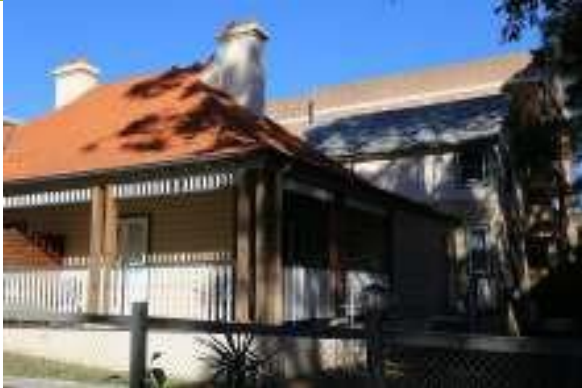
Detail of rear extension.
