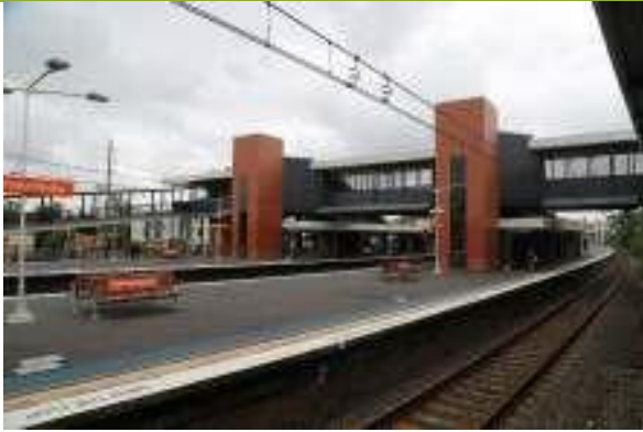
Overview of footbridge.
