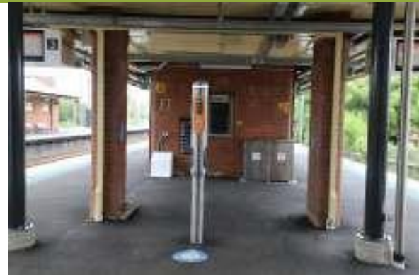
View of platform building from bottom of footbridge stairs.
