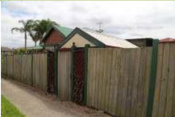
Boundary fence visible from Bennet Street.
