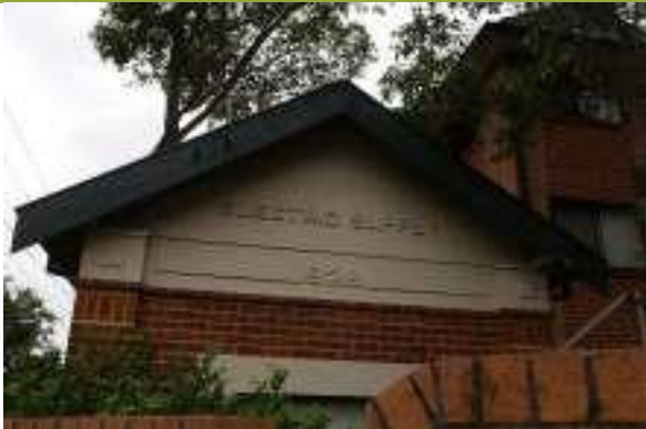
Detail of gable end showing 'ELECTRICAL SUPPLY 1928' relief.
