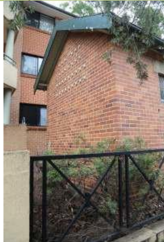
Rear elevation of substation and boundary fence.
