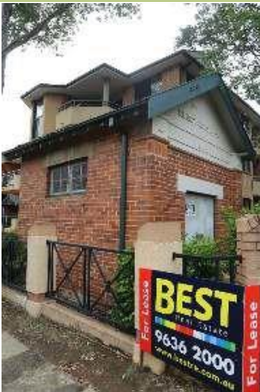
Overview of substation showing front and side elevations, as well as the boundary fence.
