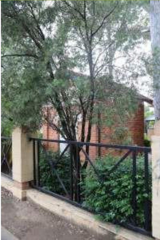
Overview of substation from the footpath along Fullagar Road.
