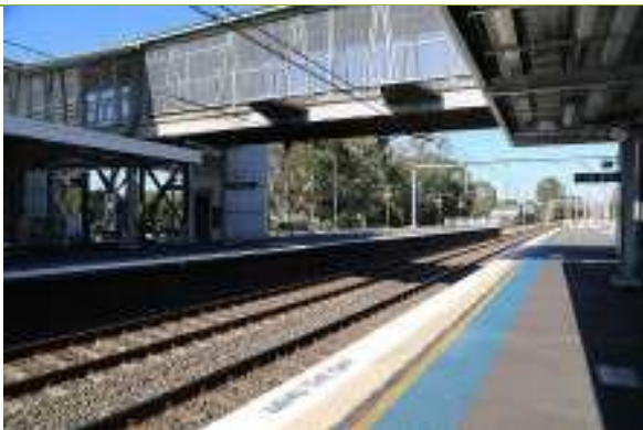
View southeast to Platform 2.
