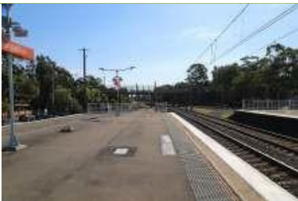
View north towards underbridge.
