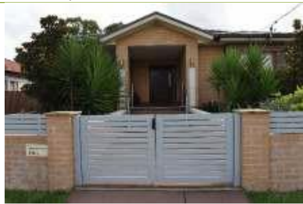
New dwelling at 278 Clyde Street.
