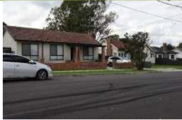
Streetscape view, Chiswick Road.
