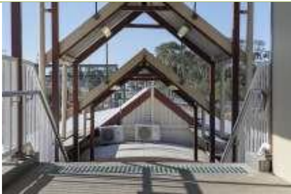
Platform canopy leading down to platform from footbridge (Source: NSW Office of Environment and Heritage, Railcorp S170 Listing Sheet for Regents Park Railway Station Group).
