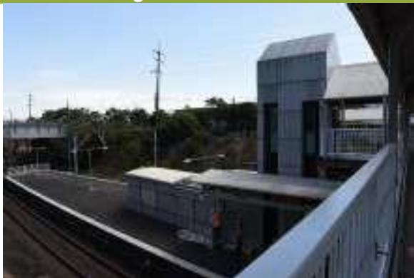
Platform footbridge and modern lift.
