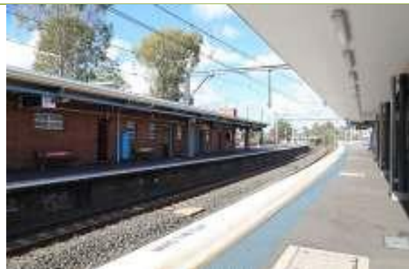
Station building as view from the opposite platform.
