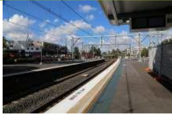
View south east along both platforms.
