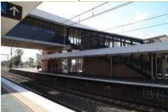
Footbridge concourse and station building from platform.
