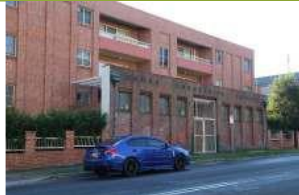
View of façade from Dunmore Street.
