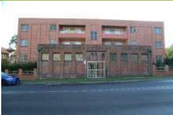
View of façade from Dunmore Street.
