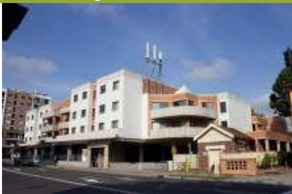
Electricity substation as it is situated on Merrylands Road.
