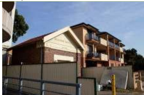
Substation showing development to the north.
