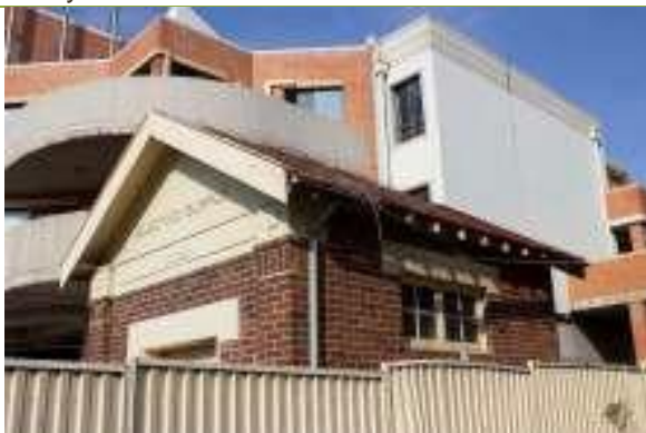
Front façade and southern elevations of substation.
