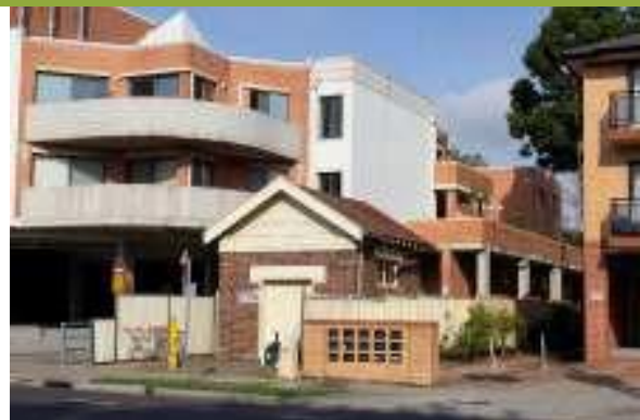
Electricity substation showing medium-density development to the south.
