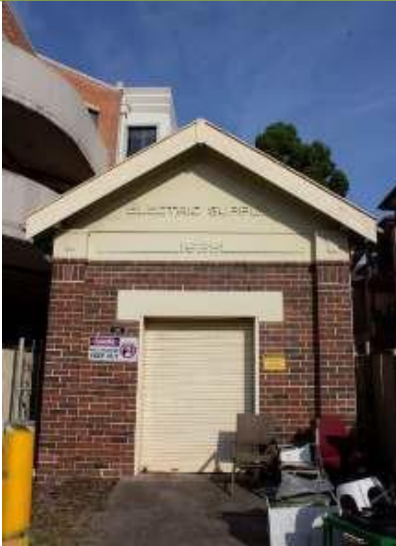
Front façade of Electricity substation.
