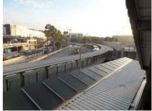
Overview of Merrylands Railway Station.
