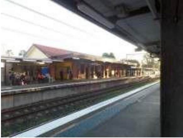
View to Station Building.
