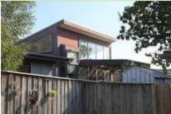
View to rear extension of cottage.
