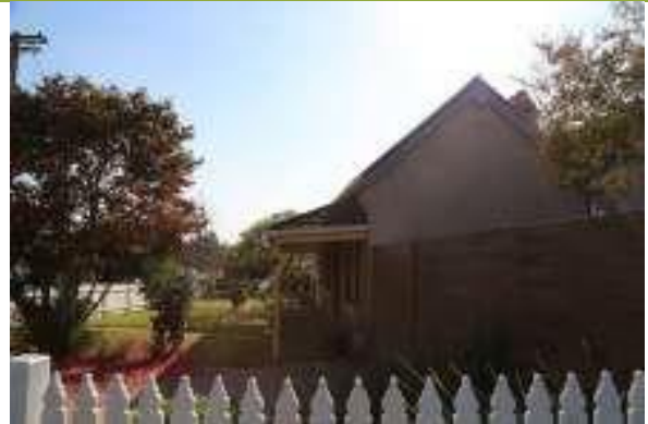
View to front of property from Kooba Street.
