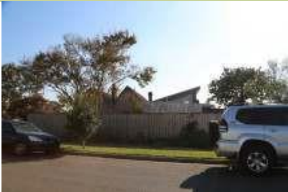
Southern elevation showing rear extension. Viewed from Kooba Street.
