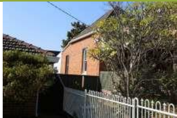
Northern elevation of cottage.
