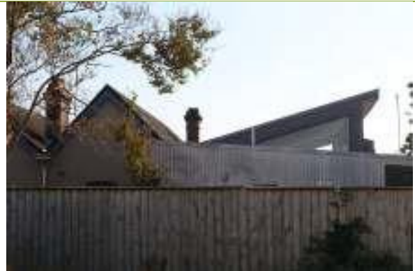
View to southern elevation.
