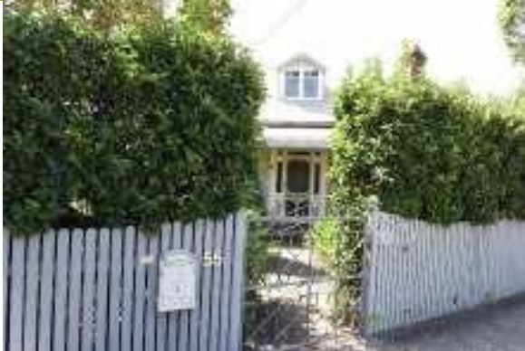
View of front façade and fencing of cottage.
