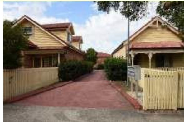
Overview of dwelling and rear subdivisions
