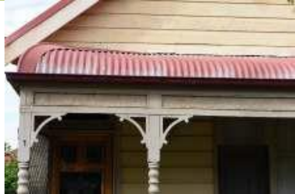
Detail to verandah.
