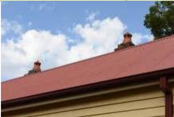
View of roof elements.
