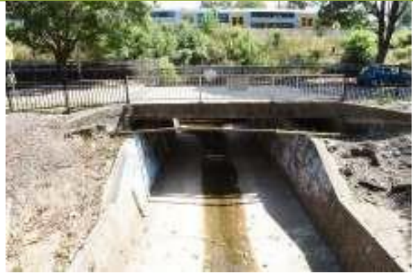
Haslam's Creek Stormwater Drain.
