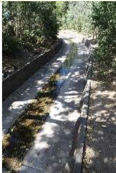
Channel of Haslam creek Stormwater Drain.
