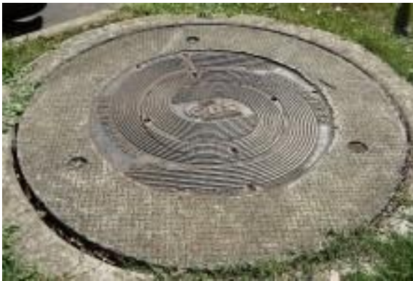
Haslam Creek Stormwater Drain.
