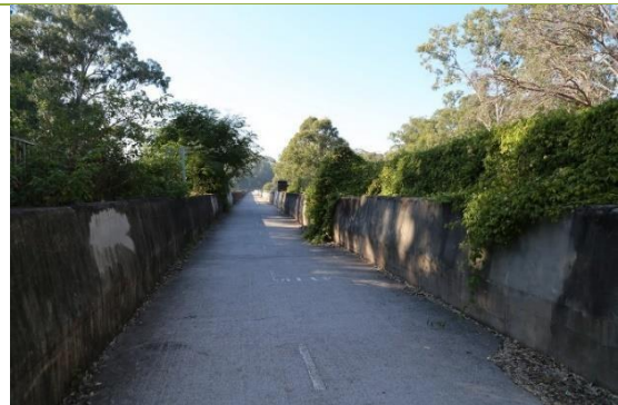
The Boothtown Aqueduct.
