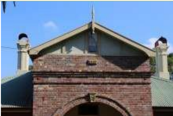
View to front facing gable.
